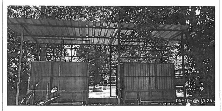
There are two compost pits each of size 5'X4'X4' an additional height of 1' above the ground is provided to make it compatible and aerated, also the possibility of rodents damaging the structure is taken care of, each pit has a capacity of 3 tonnes and it has a lid of MS steel with MS net and both the pits are being covered by a shed of 0.5 mm thick steel with coating against corrosion.
